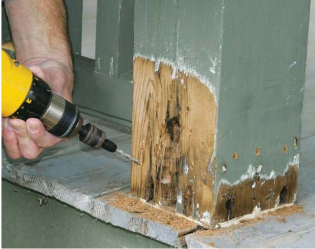
Figure 3. Drilling a series of small holes around the perimeter of a rot-damaged crevice (left) makes it possible to inject epoxy consolidant deep into the wood. To fully saturate the damaged area, the author alternates between squirting consolidant into the holes and brushing it on the surface (below).
