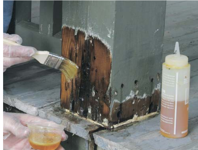
Figure 3. Drilling a series of small holes around the perimeter of a rot-damaged crevice (left) makes it possible to inject epoxy consolidant deep into the wood. To fully saturate the damaged area, the author alternates between squirting consolidant into the holes and brushing it on the surface (below).
