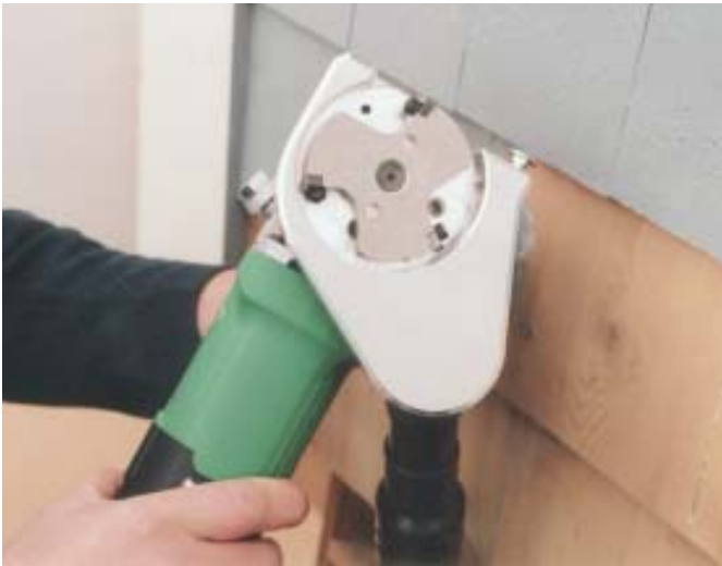
Figure 7. The Paint Shaver grinds off paint but captures almost all of it in an attached vacuum (left). The Silent Paint Remover uses low-level infra-red heat to loosen paint without releasing lead paint fumes (below).
