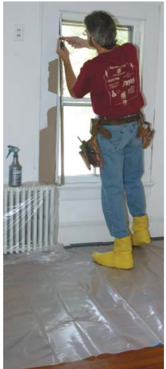
Figure 6. For a job that might disturb only a small amount of lead paint, you just need to cover the floor with a sheet of 6-mil plastic that extends 5 feet away from the work area. Plastic shoe covers keep dust off and improve traction on the slippery surface.
