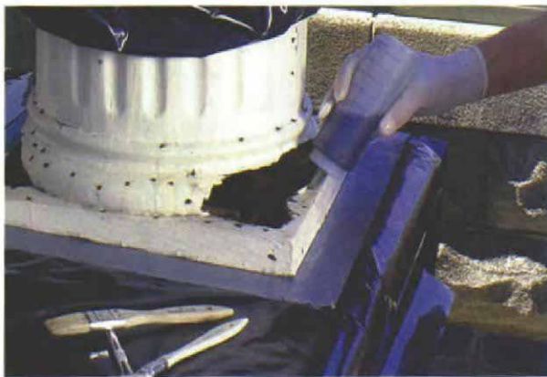
Brushed-on epoxy consolidates exposed wood. In addition to being injected, consolidant is brushed onto exposed wood until it no longer soaks into soft wood.
