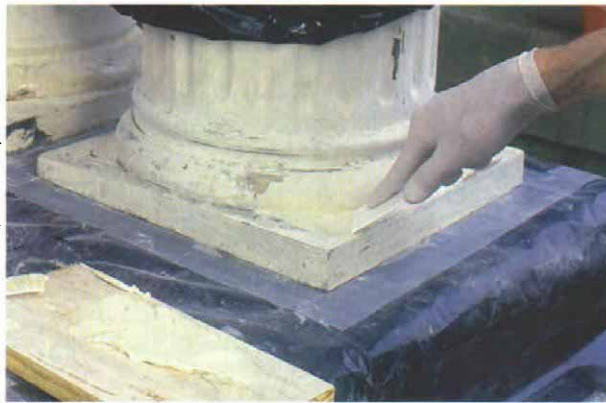
Woodworking tools also handle epoxy. Cured epoxy can be worked like wood. A chisel and a Surform plane rough out the shape, and sandpaper does the smoothing.
