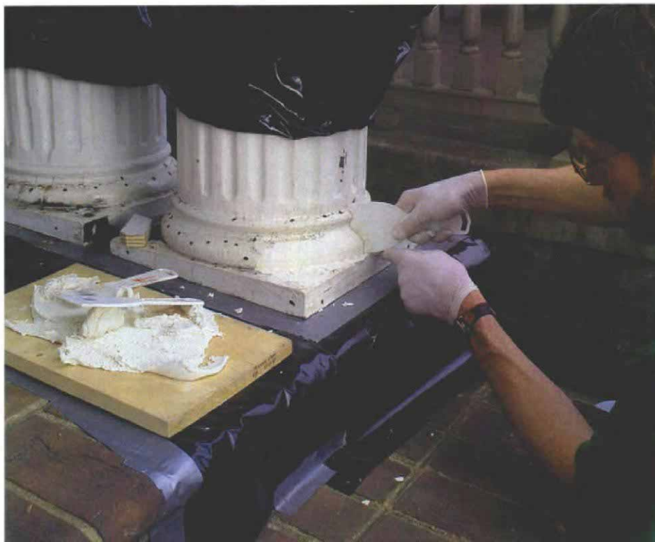
A homemade tool for re-creating odd shapes. Irregular profiles such as the fluted bottoms on these columns can be molded using a plastic putty knife with the shape cut into the blade.
