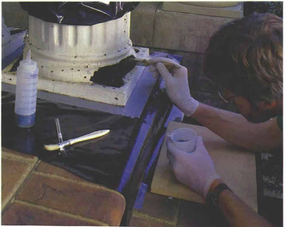
Brushed-on epoxy consolidates exposed wood. In addition to being injected, consolidant is brushed onto exposed wood until it no longer soaks into soft wood.
