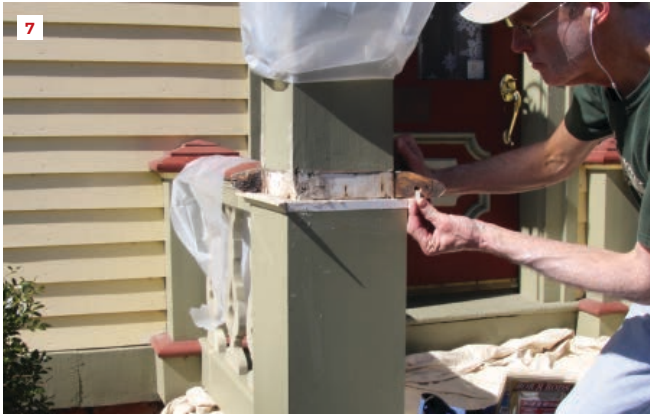
Before the miters are assembled, the author drills a hole and inserts a Bor8Rod that will provide an extra measure of insurance against rot (7).
